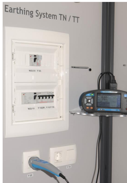
Figure 2-13: Measuring Z_{Loop} in the Application Trainer with the schuko commander
