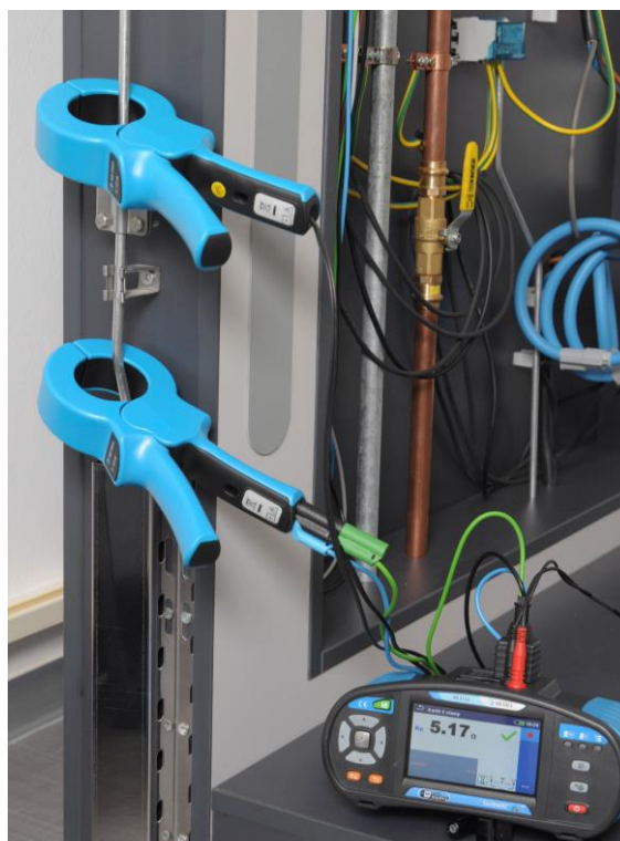
Figure 2-50: Lightning system testing
