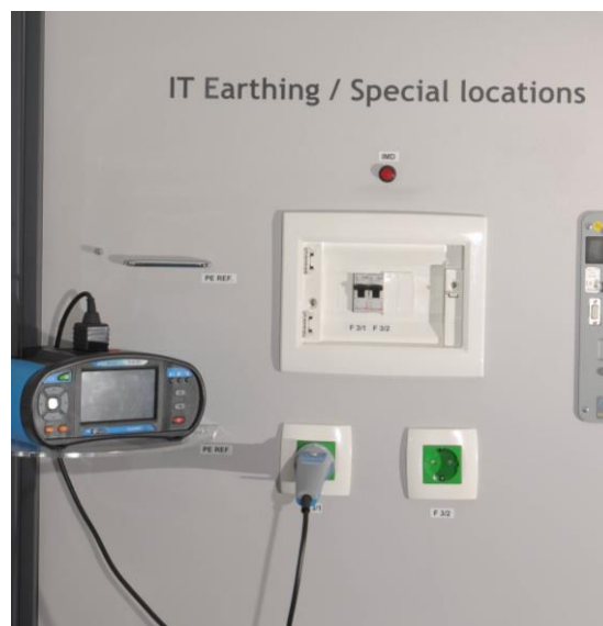
Figure 2-4: Measuring Z_{Line} in the Application Trainer with the schuko commander on an IT system
